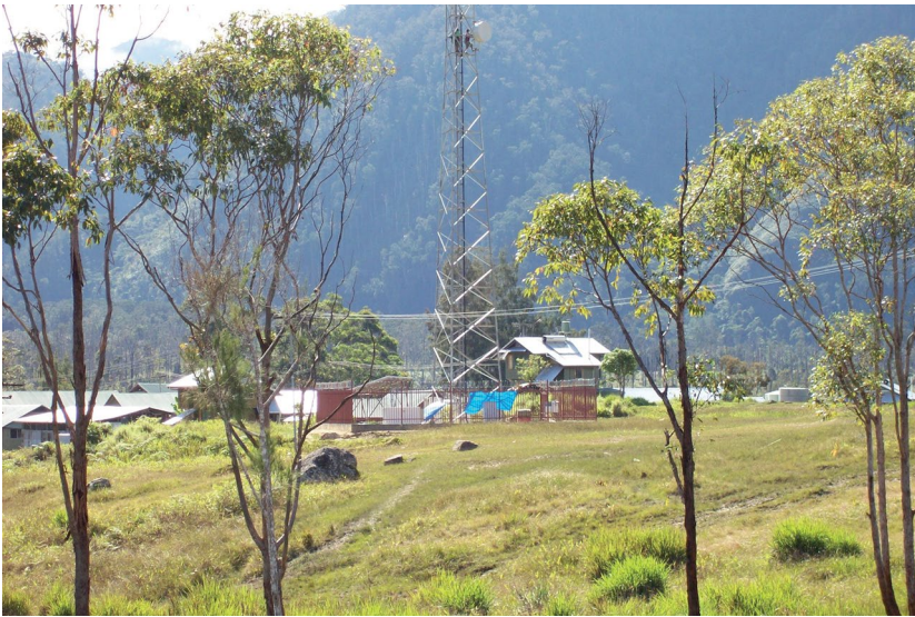
Figure 12. Digicel tower being completed, Telefomin
