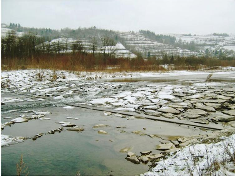
**Fig. 5.9** Ramp—close to nature structure used in mountain rivers
