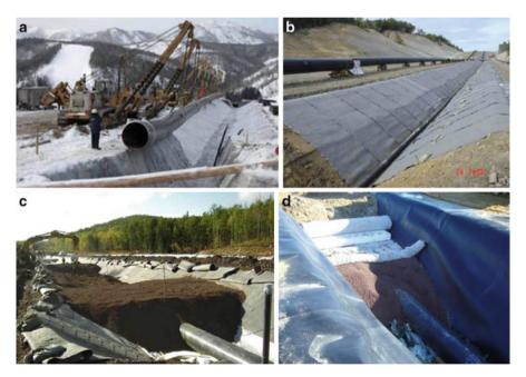
**Fig. 10.9** Some pictures during construction of the special trenches. (a) Pipeline lowering in of the special trench. (b) Detail of sub-trench HDPE drainage pipe. (c) Backfilling of wide trenches with LECA (LBM). (d) Backfilling of narrow trenches with LECA (LBM) (Mattiozzi and Strom 2008; Vitali 2014)
