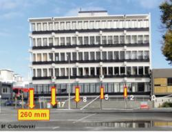
**Fig. 13.22** Example of significant tilting and differential settlement in buildings in the CBD after the 22 Feb 2011 Canterbury Earthquake (From Giorgini et al. 2012, 2014)
