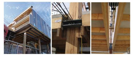
**Fig. 13.30** College of Creating Arts – MacDiarmid Building, Massey University, Wellington, New Zealand. Post-tensioned timber (Pres-Lam) frames in the transverse directions with horizontal U-Shape flexural plate dissipaters on the first floor and Post-tensioned concrete (PRESSS) walls in the longitudinal direction (Structural Engineers: Dunning Thornton Consultants)
