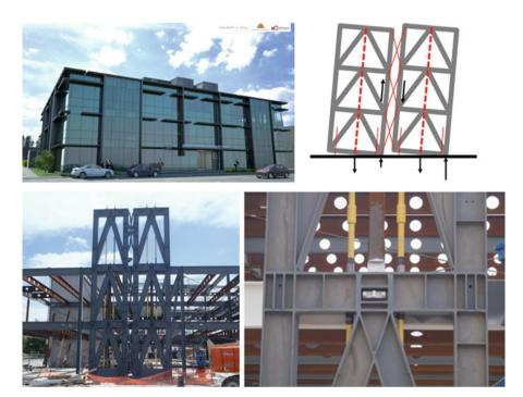
**Fig. 13.34** Forté Health Medical Centre, three storey building with over 5,000 m<sup>2</sup> of specialist medical facilities. Post-tensioned steel rocking coupled 'walls' (or braced-frames) in both directions, combining hysteretic and viscous dampers in parallel for "an advanced flag-shape" system. *Bottom right*: secondary interior moment-resisting frames implementing a sliding hinge joint beam-column connection solution
