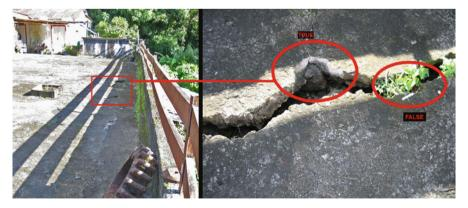
**Fig. 16.6** False declaration by the inhabitants of terrace collapse (Les Saintes earthquake 2004). In fact the terrace is not collapse and it's only an increase of existing crack created by an amplification of differential collapse. We can see on the right picture the presence of vegetation in the crack, meaning the age of this damage
