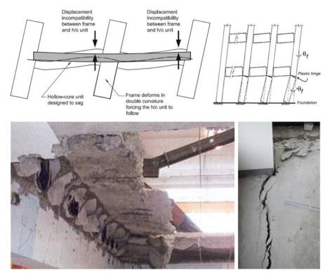
**Fig. 13.14** *Top*: Example of vertical (*left*: after Matthews et al. 2003) and horizontal (due to beam elongation effects) displacement incompatibility (*right*: after *fib* 2003). *Bottom*: collapse of floor units in an 3-D experimental superassemblage test (*left*: after Matthews et al. 2003) and extensive damage to the diaphragm topping of precast concrete floors in a multi-storey building following the 22 Feb 2011 Canterbury Earthquake (*right*: after Kam et al. 2011)
