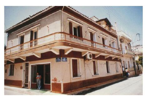
Fig. 16.8 Unreinforced masonry with RC floors, grade of damage 3, in Greece 1995 (Grünthal 1998, EMS-98 scale)
