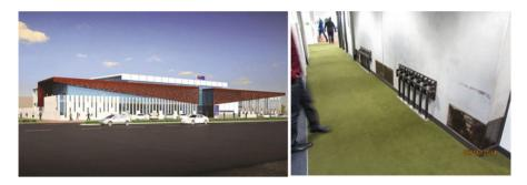
**Fig. 13.26** Police Station in Rotorua. Post-tensioned concrete (PRESSS) walls with external & replaceable dissipaters in both directions (Structural Engineers: Spiire)
